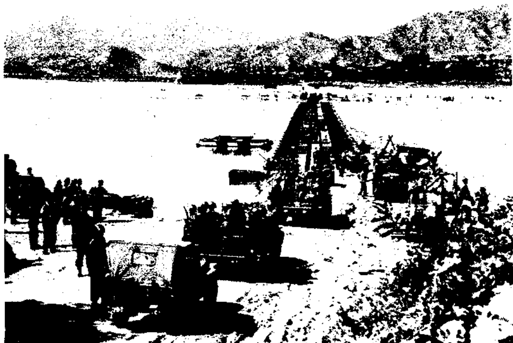
Pontoon treadway bridge across the Naktong, built in thirty-six hours.
