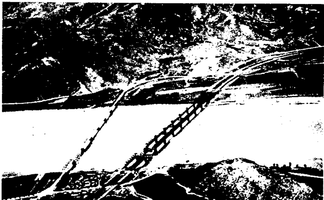
Highway and railway bridges over the Nakdong near Waegwan.
