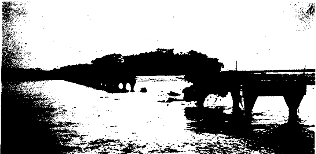
A Kum River bridge was destroyed by US troops before withdrawing to the south bank of the Kum on 12-13 July.
